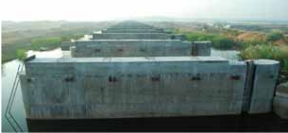
Fig. 3.9.1: Cauvery - Gundar Link – Barrage Construction
