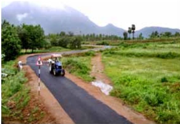
Fig 4.4: Link Road- PMGSY
