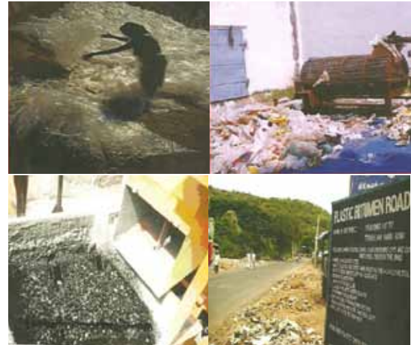
Fig. 15.2.9: Re-laying of Roads with Plastic Waste
