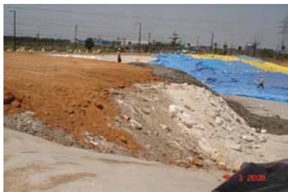
Fig. 15.2.10: Hazardous Waste Management , Gummidipoondi
