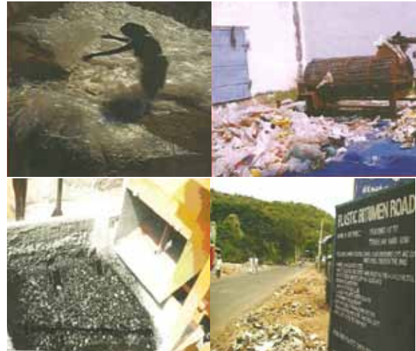
Fig. 15.2.9: Re-laying of Roads with Plastic Waste
