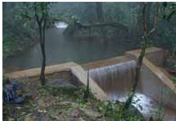
Fig.15.3.8: Water Conservation Works Under HADP
