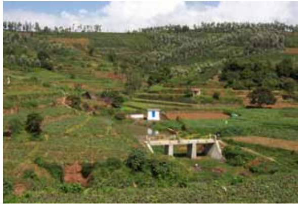
Fig.15.3.2: Provision of foot bridge in rural Ooty
