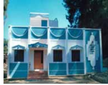
Fig.15.3.7: Construction of farmers training centre in Ooty
