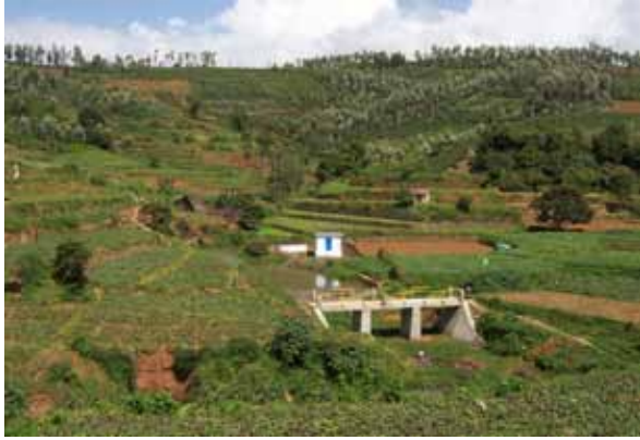
Fig.15.3.2: Provision of foot bridge in rural Ooty
