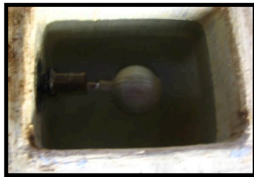
BALL FLOAT MECHANISM
