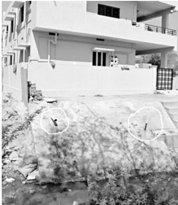
Health hazard: Wastewater from houses flowing into the distributory canal of the
