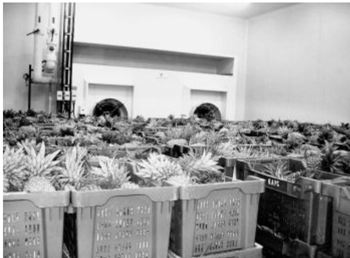
Farm fresh:The new cold storage facility at Muvattupuzha. —
