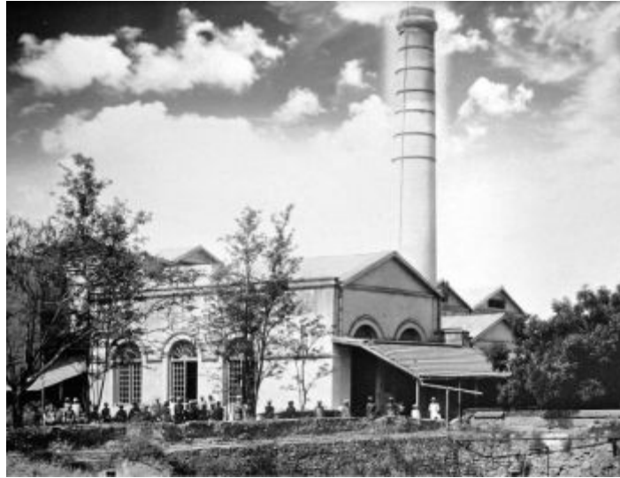
The Coimbatore Spinning and Weaving Company Limited in 1888.
