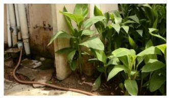
The process of recycling grey water using canna plants is cost-effective and simple. A filtering system at a residential complex in T.Nagar. — Photo: K.V.Srinivasan
