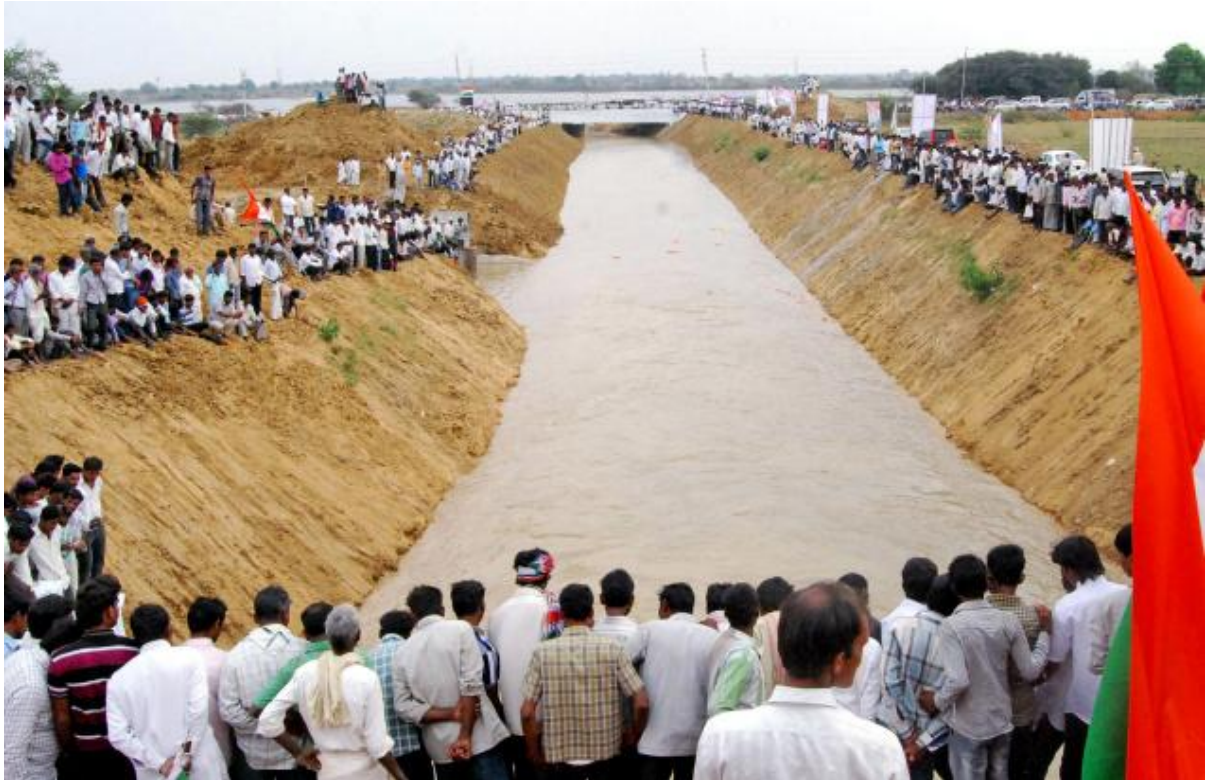
Big day:Water being released from the Singoor project to a canal after it was formally inaugurated by Deputy Chief Minister C. Damodar Rajanarasimha, in Medak district on Thursday.- PHOTO: MOHD ARIF
