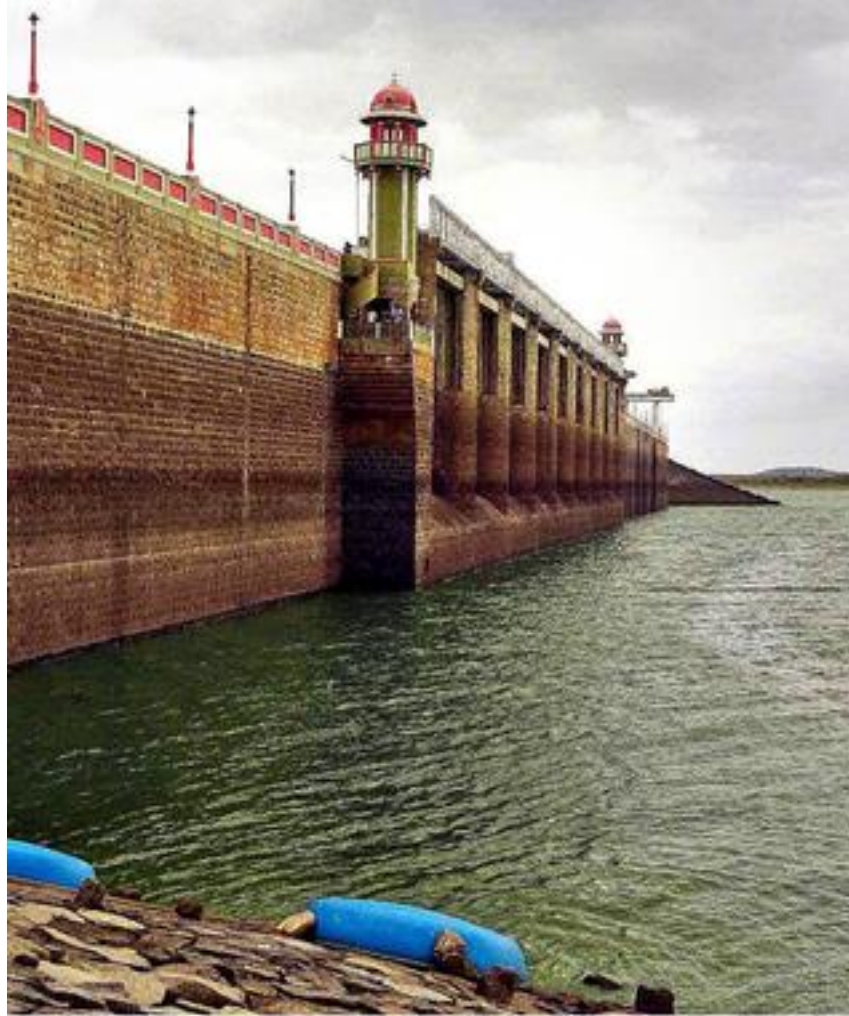
A view of Bhavani Sagar Dam reservoir in Erode.
