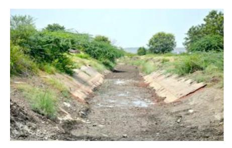
The right bank canal of the Bennethora Major Irrigation Project has been damaged in several places with missing concrete linings allowing seepage of water into the agricultural fields, thereby damaging standing crops, in Kalaburagi district.
