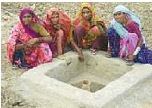
» Constructed Drainage System
