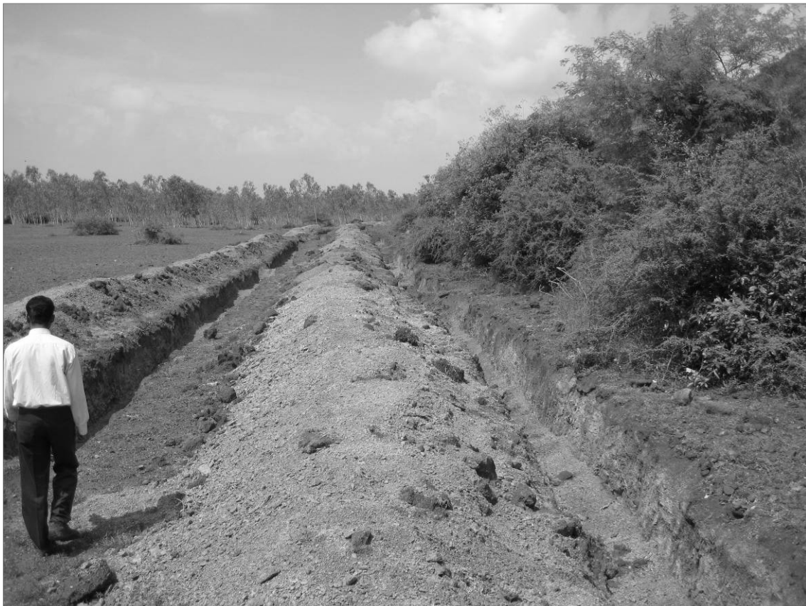
Figure 4 Trenches in Arapedu.
