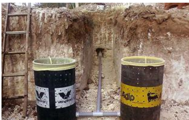
The device developed by S. Sivakumar to increase rate of recharge in borewells.
