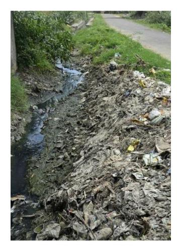
Drainage water flowing through an incomplete channel in front of the SOLAI farm in Vandranthangal village near Katpadi. The point up to which the channel has been constructed and left incomplete can be seen at the top left of the picture —Photo: C. Venkatachalapathy
