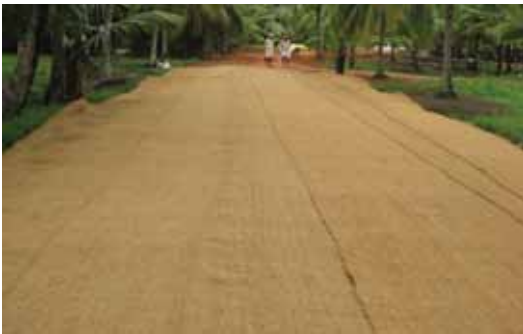
Placing of coir geo textile and surfacing of road Mangalabharathy SN Kadavu road in Haripad
