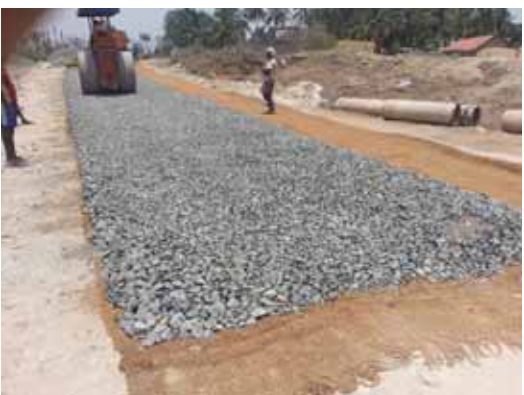
LAYING AND ROLLING OF AGGREGATE
