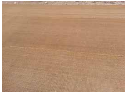
Coir geo textile ready for sub base
