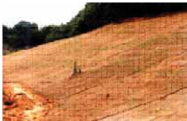
Eroded bank and Geo textiles laid on leveled bank of reservoir, Kakkayam
