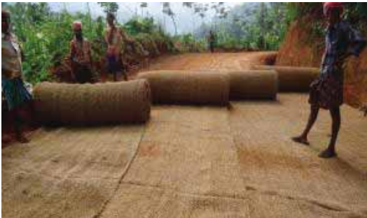
Keep the rolls adjacent and find out the overlap that can be given
