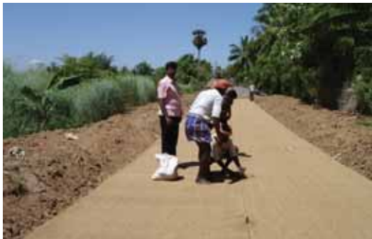
Fixing of coir geo textiles
