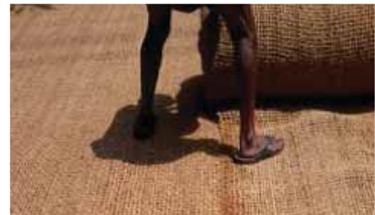
Roll out second& third rolls while maintaining required overlap
