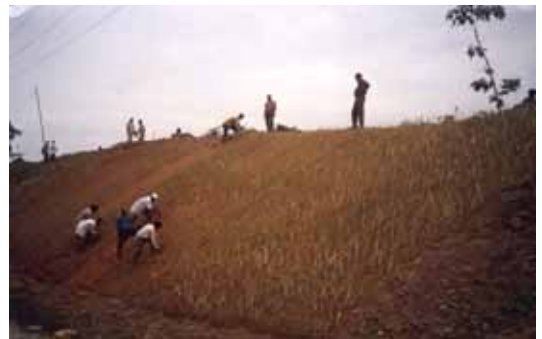
Protection of Road Embankment, Silchar, Assam
