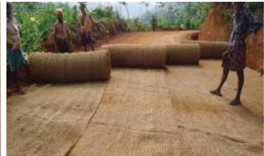
Roll out first roll with one of edges as reference
