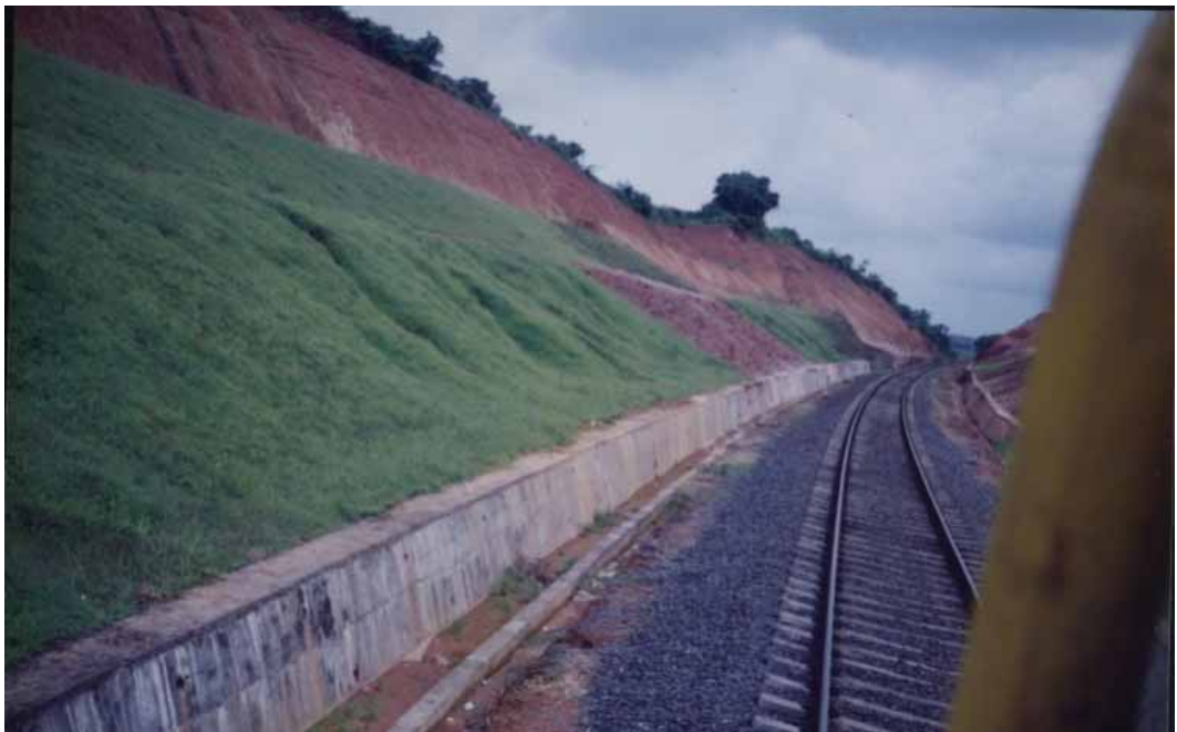
Protection of railway embankment, Konkan railway
