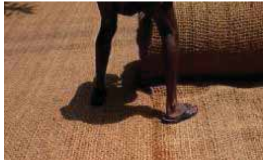
Roll out second & third rolls while maintaining required overlap
