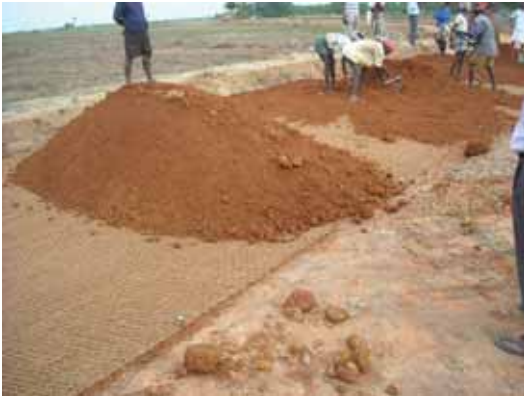
Laying of Sub base over coir geo textiles
