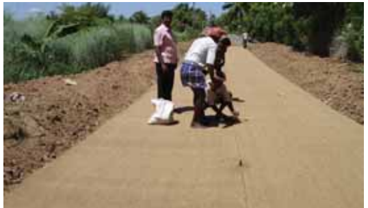
Fixing of Coir Geo textile
