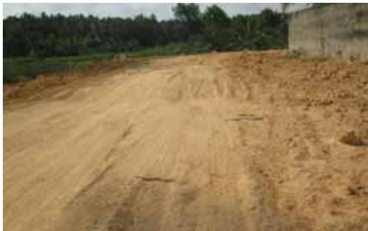
Before laying coir geo textiles
