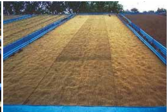
Leveled slope laid with coir geo textiles
