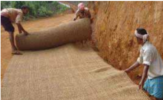
Roll out second & third rolls while maintaining required overlap
