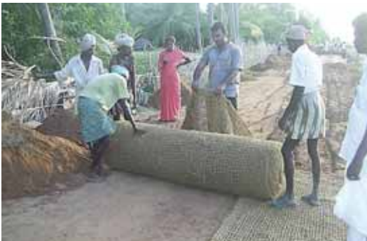
Laying of Coir Geo textile
