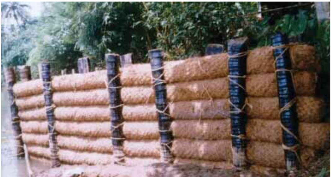
Cocolog laid on the banks of Pampa river for preventing soil erosion
