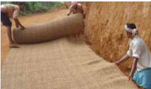
Roll out second& third rolls while maintaining required overlap
