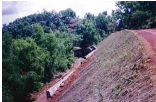
Stabilised road embankment
