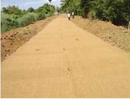
Coir geo textile ready for sub base
