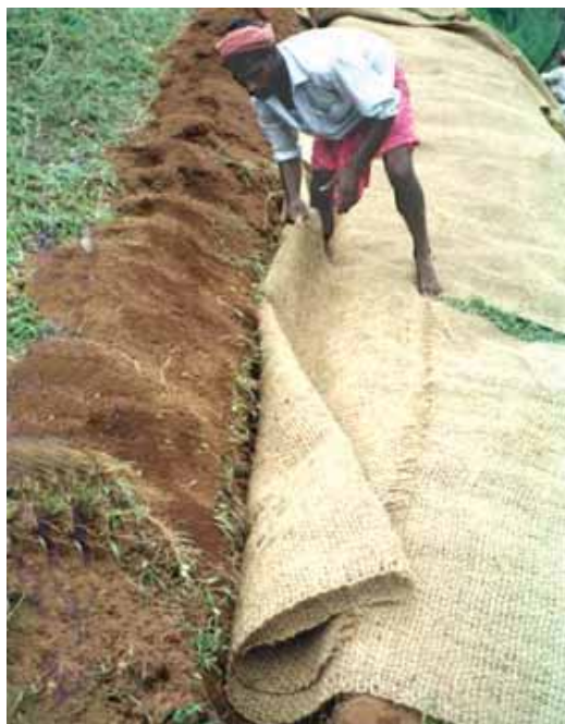
Laying of coir geo textiles in trench
