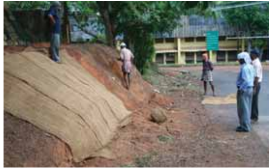
Stabilization of Embankment, College of Engineering, Trivandrum
