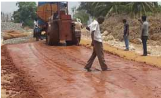
SPREADING, WATERING AND ROLLING OF GRAVEL, LAYING OF PMC
