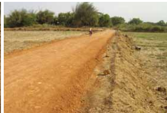
Finished Sub base Ready for Coir Geo textiles laying
