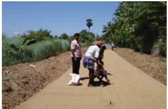
Fixing of coir geo textiles
