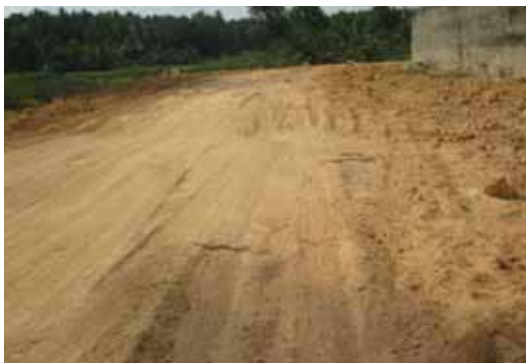
Before laying coir geo textiles
