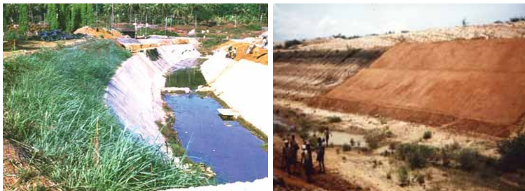
Protection of irrigation canal embankment, Muvattupuzha and Kabini canal embankment, Mysore
