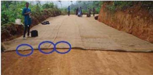
Fix the roll to the subgrade by using clamps with one metre spacing
