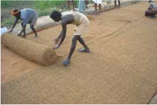
Laying of coir geo textiles
