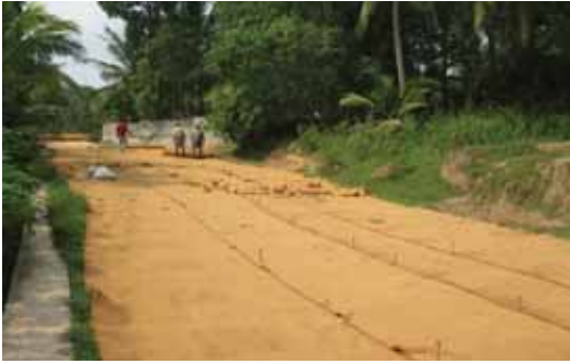
Laying of coir geo textile and Placing of soil above geo textile in Kozhinada
