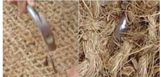
Fix the roll to the subgrade by using clamps with one metre spacing
