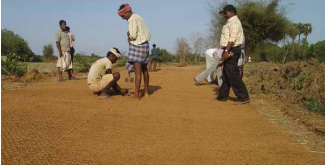
Fixing of Coir Geo textile
