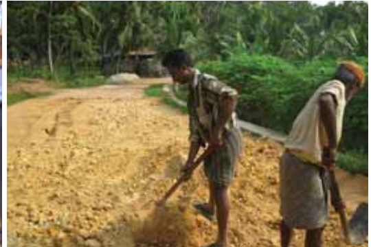
Placing of soil above geo textiles
