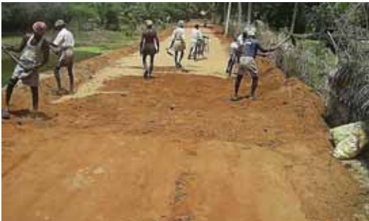
Laying of Sub base
