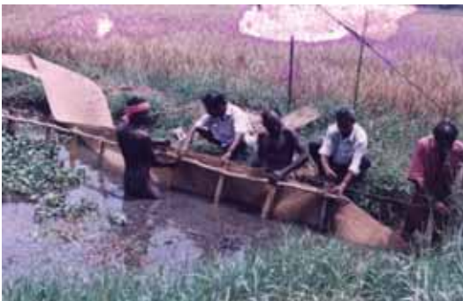
Reinforcement of Mudwall, Mankompu, Kuttanad
