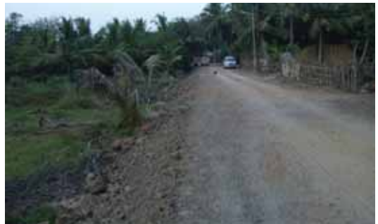
Finished Sub grade
