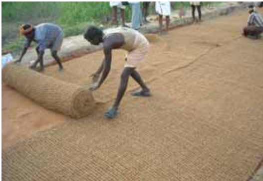
Laying of coir geo textiles
