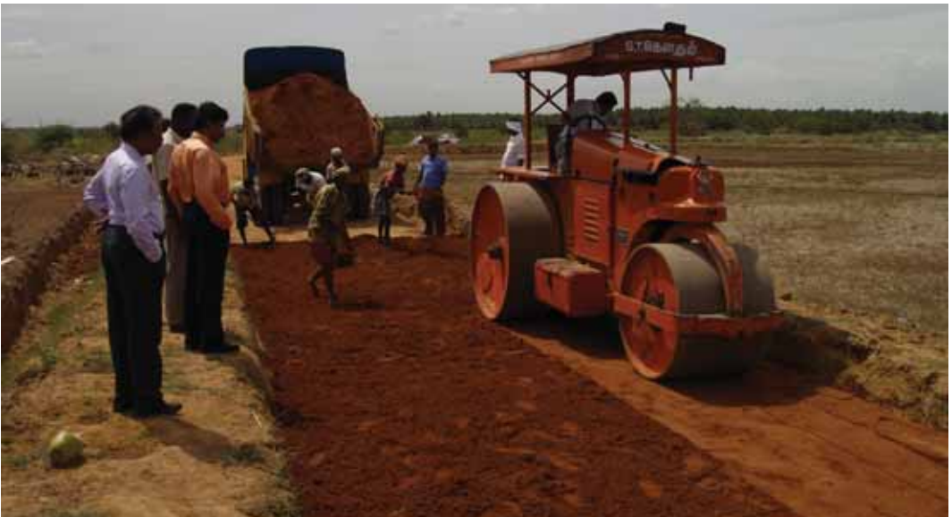
Compacting sub base with Road Roller
