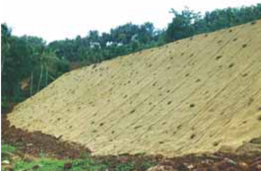
Coir geo textiles laid road embankment
