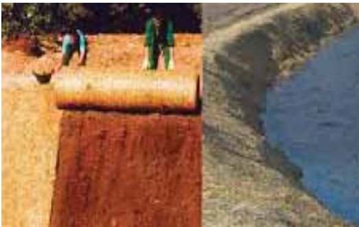
SLOPE STABILISATION OF CANAL
