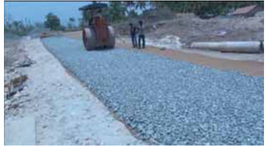
LAYING AND ROLLING OF AGGREGATE
