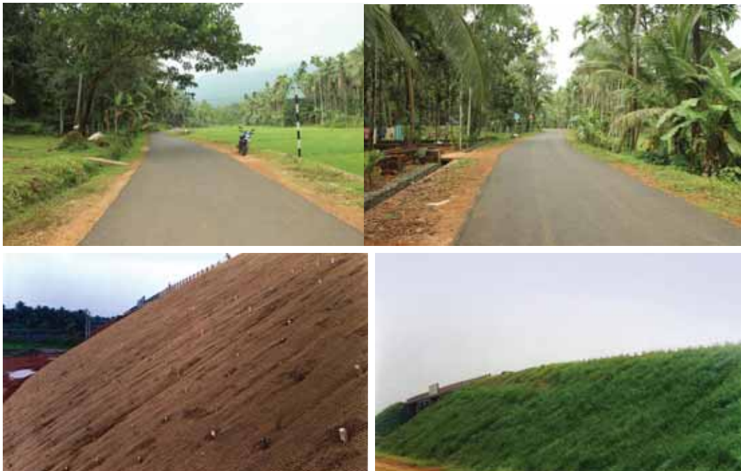
Slope Stabilisation and Growth of Vegetation, Nedumbassery Airport Approach Road
