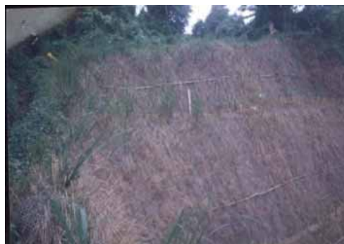
Hill slope protection
