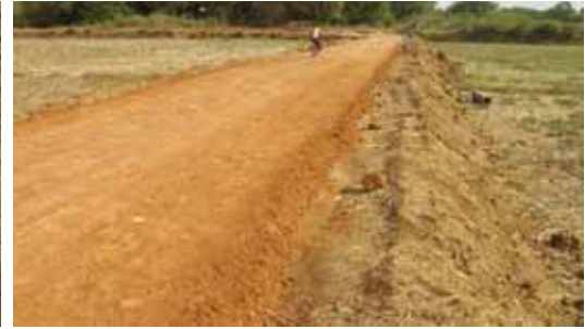
Finished sub base ready for coir geo textiles laying
