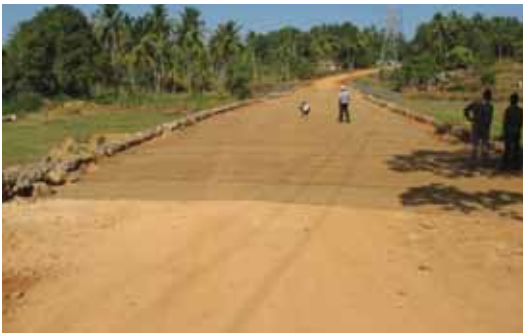
Placing of coir geo textile and surfacing of Chirakkad- Kumbakkad road (Varkala)
