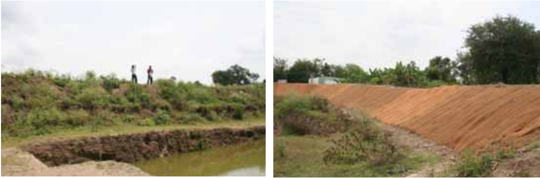
Reinforcement of rainwater harvesting pond at Thozhuthur, Kumbakonam, Tamil Nadu
