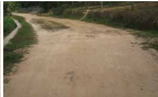
Leveled sub grade before laying coir geo textiles at Kozhinada
