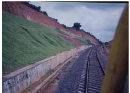
Protection of Railway Embankment , Konkan Railway
