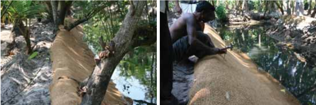
Protection of canal embankment, Arattupuzha
