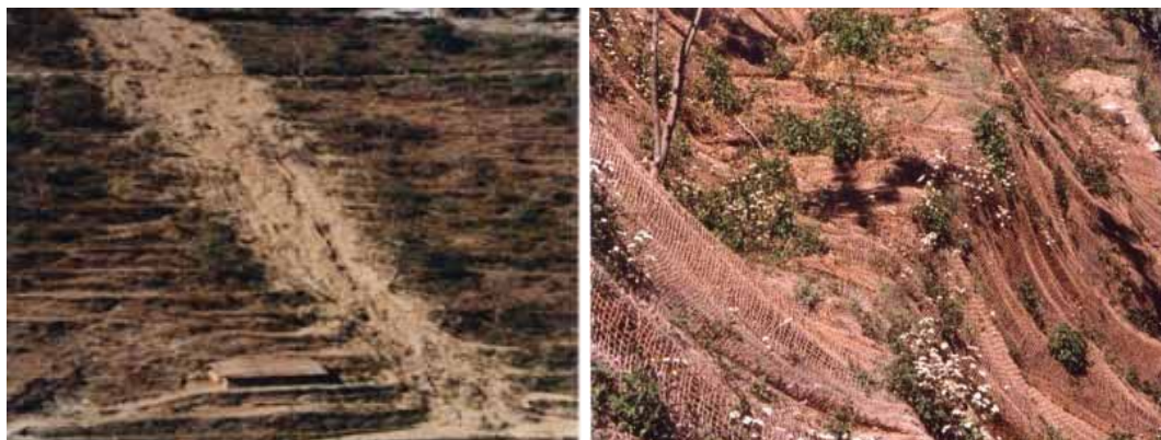
Stabilization of landslide Khandikhal, Uttarkhand
