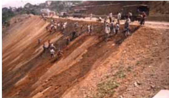
Leveling of eroded road
