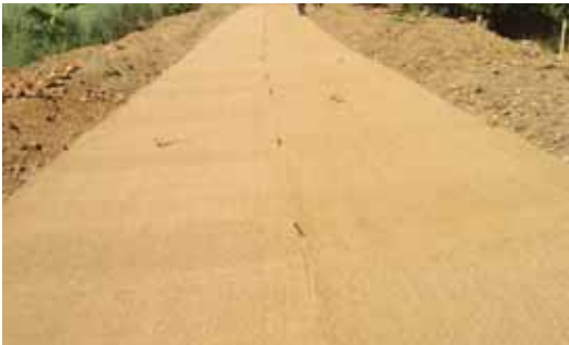
H2M8 Coir Geo textile Ready for Sub base
