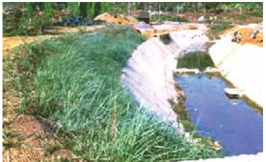
Protection of Irrigation Canal Embankment, Muvattupuza
