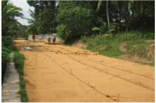
Laying of coir geo textiles
