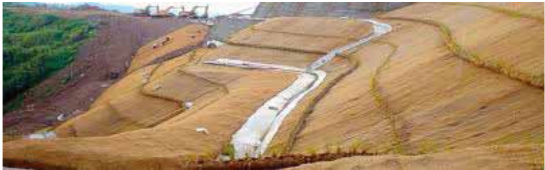
STABILISATION OF HILL SLOPES
