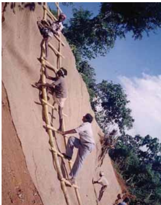
Laying of coir geo textiles
