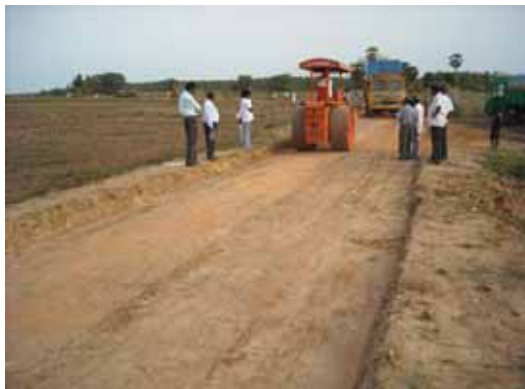
Finished Sub grade
