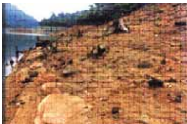
Eroded bank and Geo textiles laid on leveled bank of reservoir, Kakkayam
