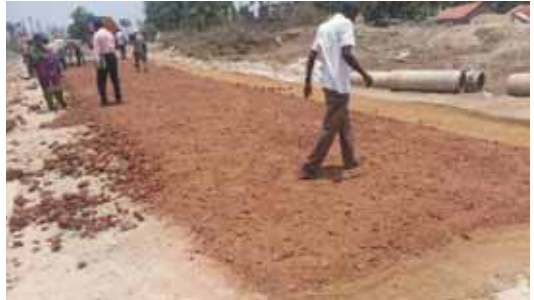
LAYING AND ROLLING OF AGGREGATE
