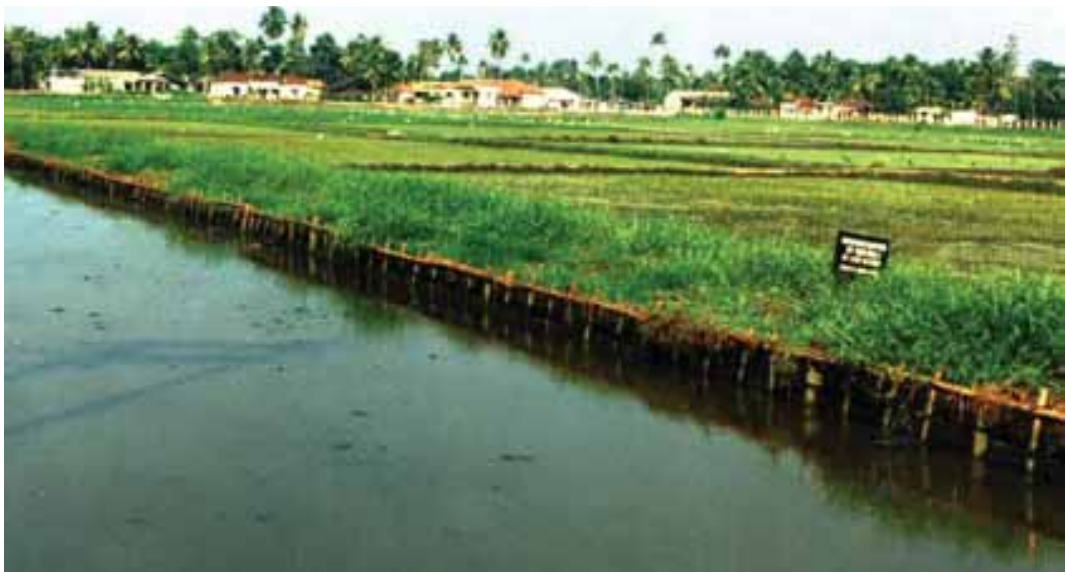
Reinforcement of mudwall,Monkompu,Kuttanadu
