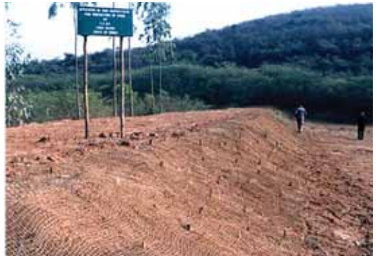
Erosion Control of Embankment, Tapovan, Gwalior
