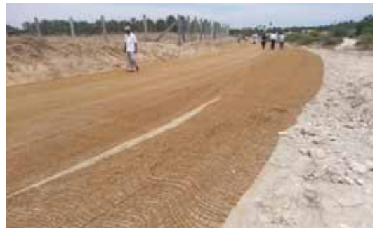
Laying of coir geo textiles
