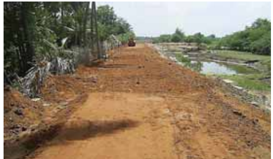
Compacting Sub base with Road Roller
