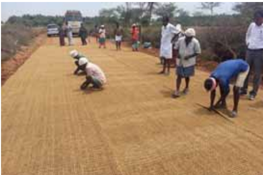
Fixing of coir geo textiles
