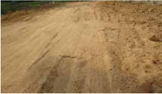
Before laying coir geo textiles
