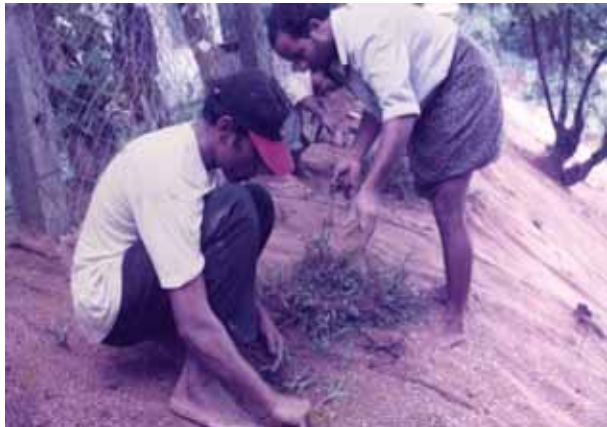
Laying of coir geo textiles and planting of grass on laid coir geo textiles on Periyar river bank
