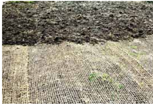
Spreading of coir pith over CGT
