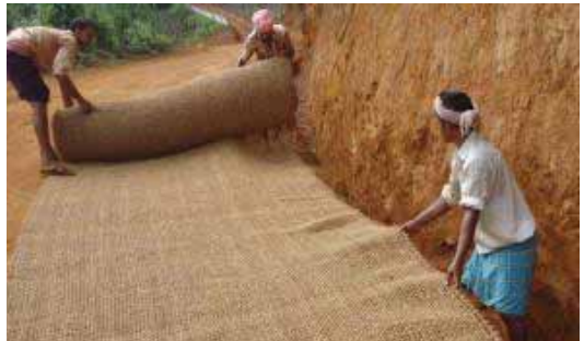
Roll out first roll with one of edges as reference
