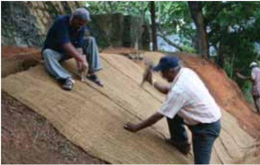
Stabilization of Embankment, College of Engineering, Trivandrum
