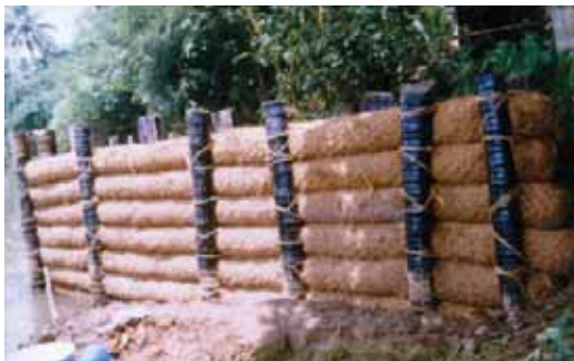
Pamba River Bank Protection
