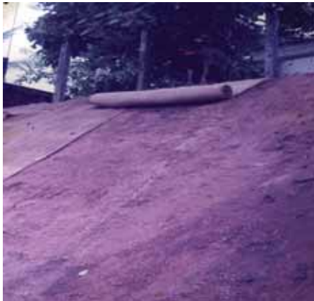
Laying of coir geo textiles and planting of grass on laid coir geo textiles on Periyar river bank
