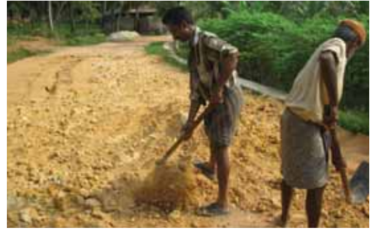
Laying of coir geo textile and Placing of soil above geo textile in Kozhinada
