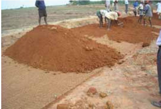
Laying of sub base over coir geo textiles
