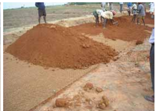
Laying of Sub base over H2M6 Coir Geo textile
