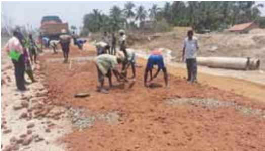
LAYING AND ROLLING OF AGGREGATE
