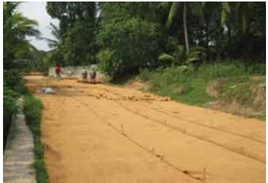
Laying of coir geo textiles
