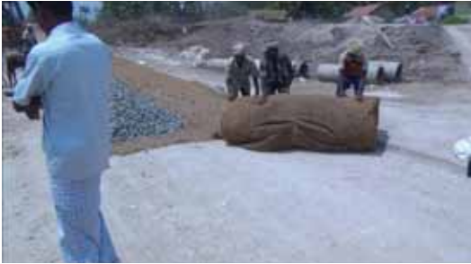
LAYING AND ROLLING OF AGGREGATE
