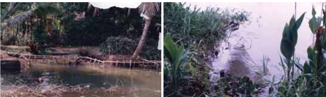
Reinforcement of stream embankment, Vellamathara, Kuttanadu
