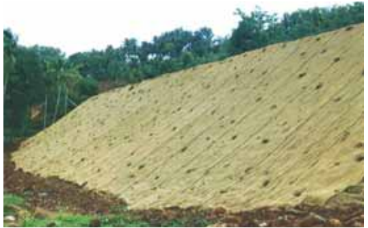
Erosion Control of Road Embankment, IIM Kozhikode
