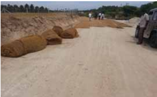
Laying of coir geo textiles
