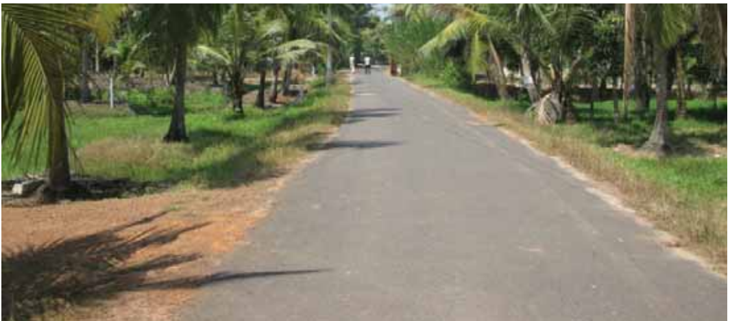
Surfacing of road
