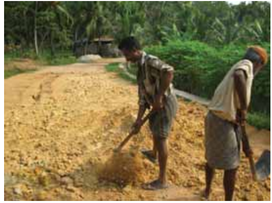
Placing of soil above geo textiles
