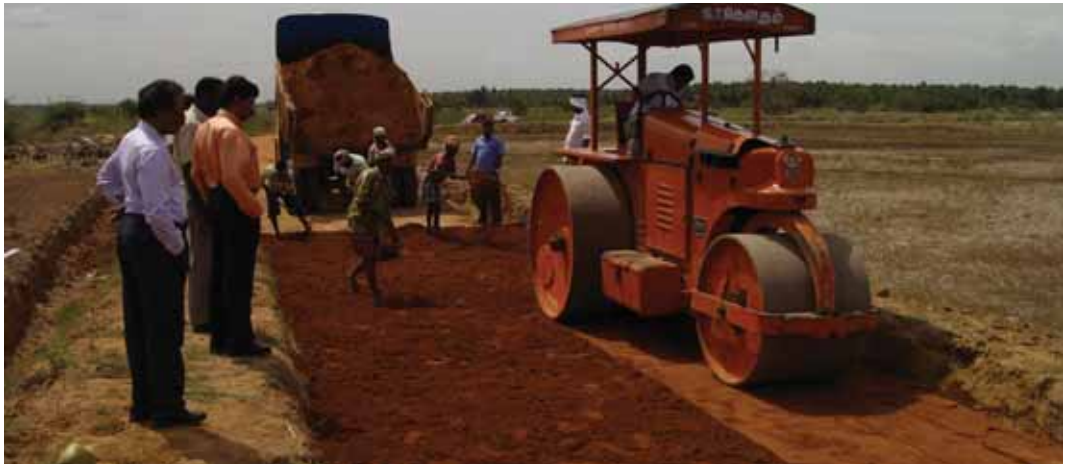
Compacting sub base with Road Roller
