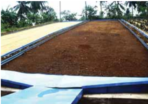
Leveled steep slope
