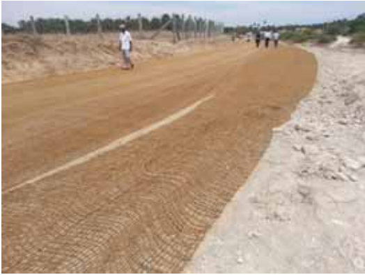
Laying of coir geo textiles
