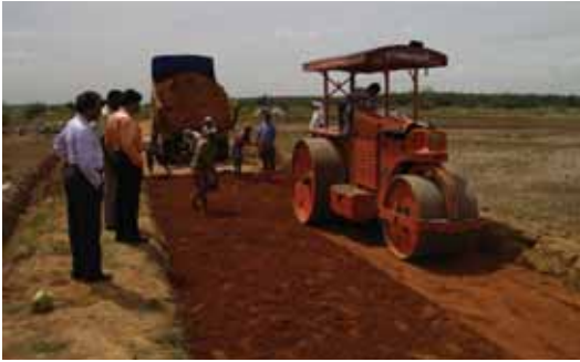
Compacting Sub base with Road Roller
