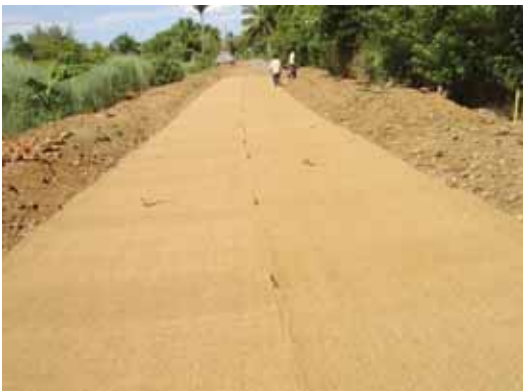
Coir geo textile ready for sub base
