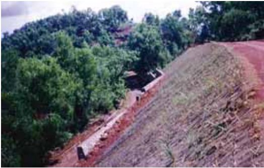
Erosion Control of Road Embankment, IIM Kozhikode
