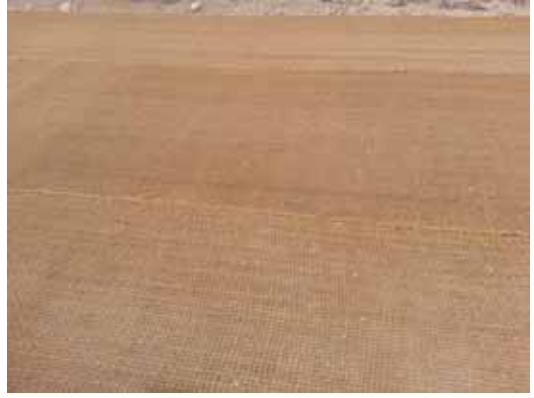
Coir geo textile ready for sub base
