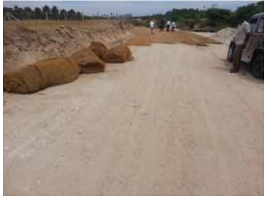
Laying of coir geo textiles
