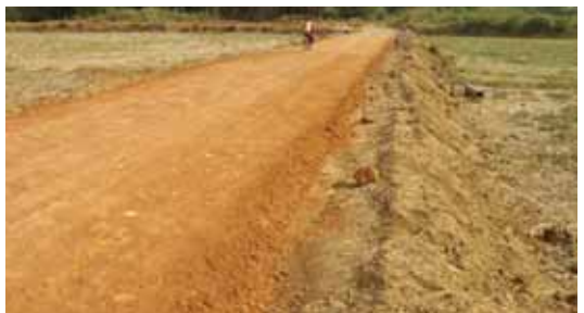
Finished Subbase Ready for Coir Geo textile laying
