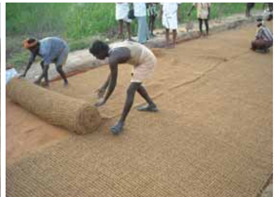
Laying of Coir Geo textile
