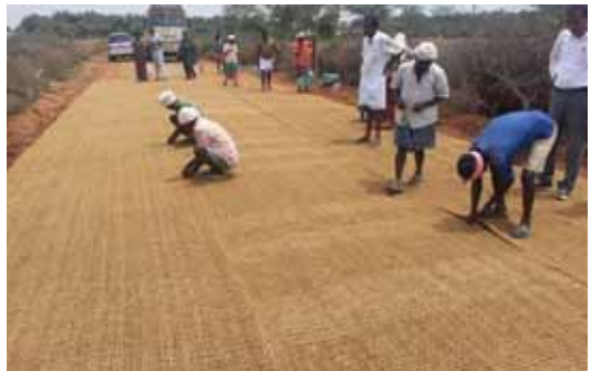
Fixing of coir geo textiles
