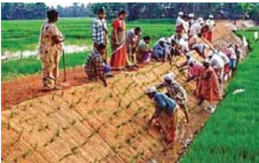
Reinforcement of unpaved road in paddy field
