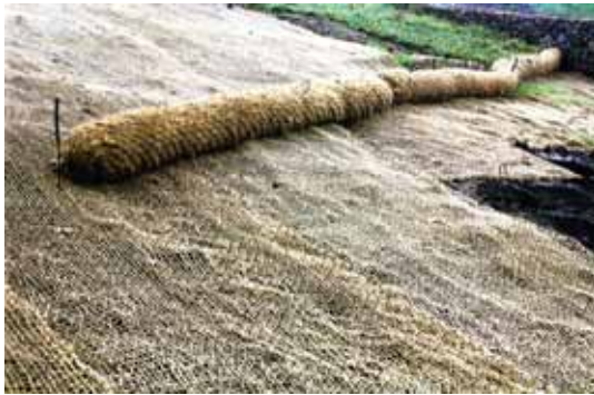
Laying of CGT over exposed rocky patches
