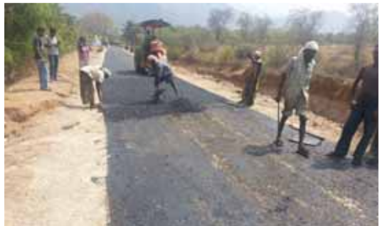
SPREADING, WATERING AND ROLLING OF GRAVEL, LAYING OF PMC
